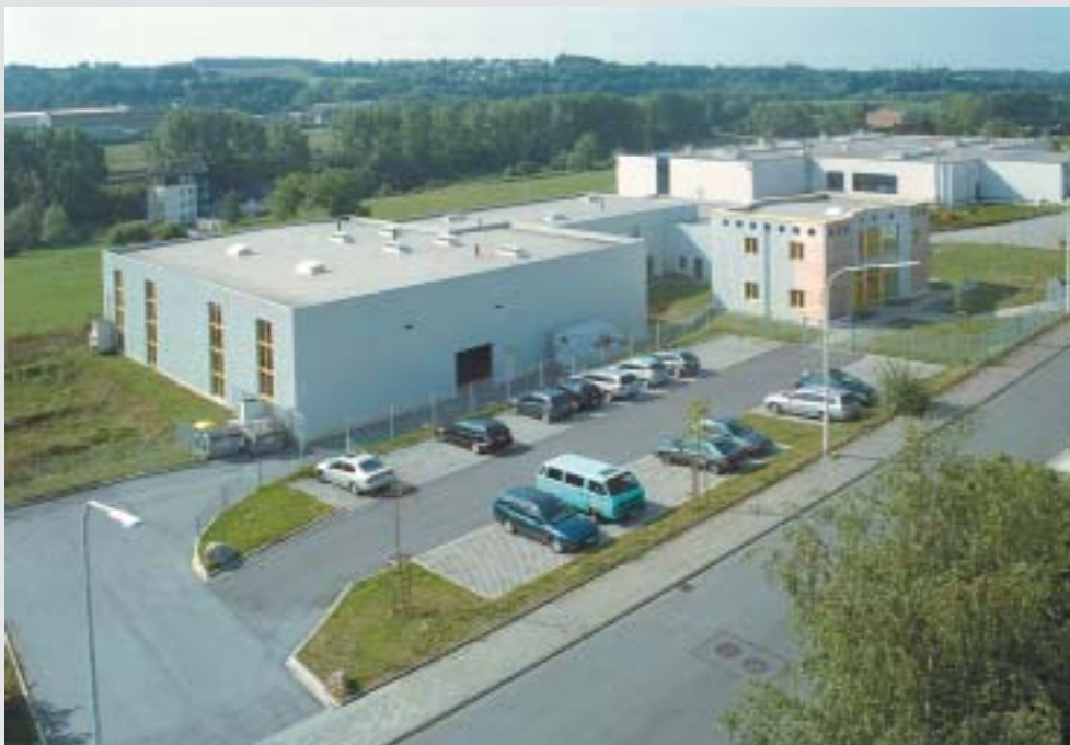
Our company buildings in Wuppertal-Vohwinkel
